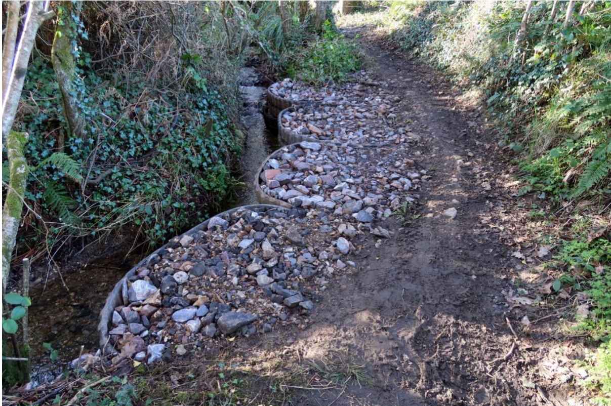
Creative use of old mini digger tracks
